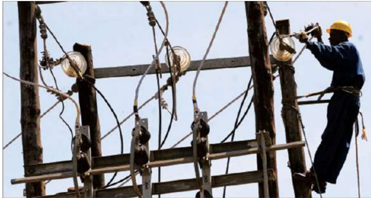
Fig. 4.6: Higher capacity transmission lines being set up
