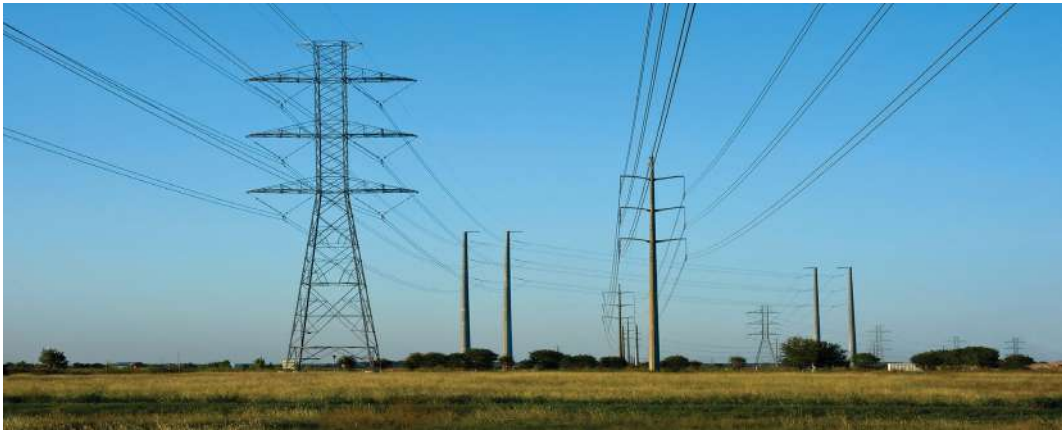
Fig. 8.15: Pylons and electricity transmission cables
