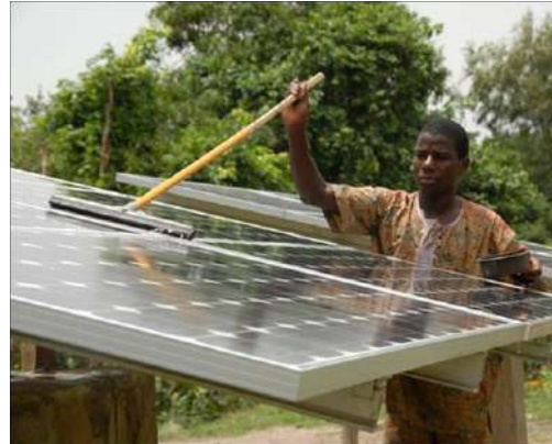
(b) Cleaning solar panel
