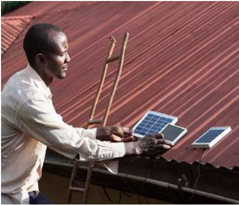
(a) Placing solar panel on the roof top
